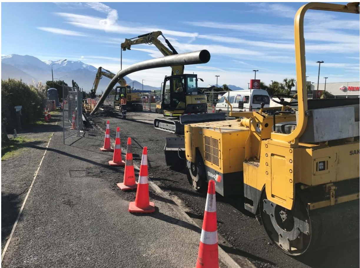
Kaikōura District Council's Beach Road sewer trunk renewal
